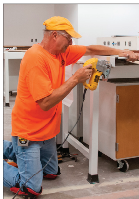
Contractor assembling tables for renovated labs
