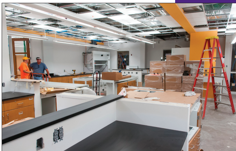
Cabinets, countertops and fume hoods being installed July 2012
